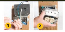
Fast, Easy Installation – Installation of each IPLC unit is estimated to take 15 minutes or less. Just remove the existing duplex receptacle, connect IPLC's colour coded wiring and attach a weatherproof cover to meet code (not included). Visit www.iplc.com for mounting options.
